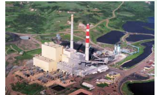
Supervisión online del Sistema ABACO de Battle River para ATCO POWER. Online supervision of ABACO system at Battle River for ATCO POWER.
