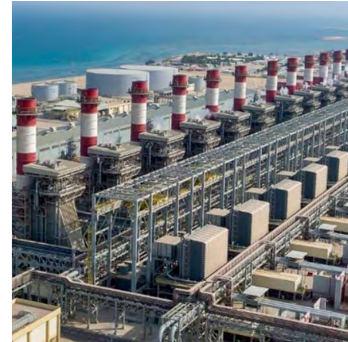
Fuente: HAJR ELECTRICITY PRODUCTION COMPANY
