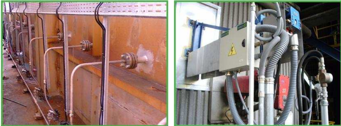
Figure 1: Advanced Monitoring Technology Sampling Probes (Options: fixed non-cooled or retractable water-cooled)
