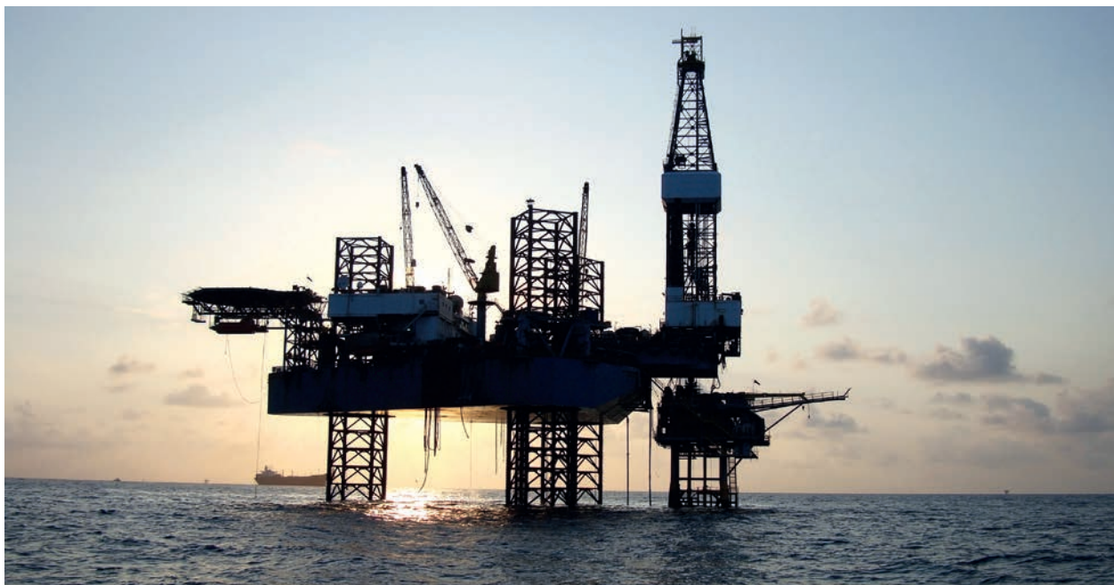
Estudios de Riesgos en Plataformas petrolíferas offshore. Risk Assessments on offshore oil platforms.
